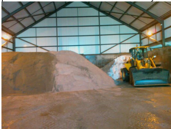
Salt Barn at Eco Depot – there is more salt in it now !
